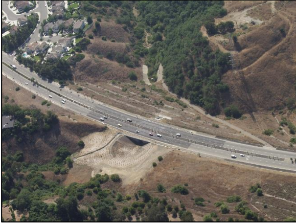
Figure 13. The Harbor Boulevard underpass as viewed from above. Image: Melanie Schlotterbeck.
