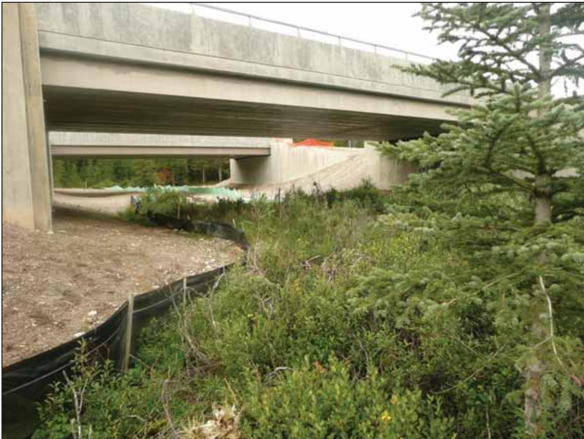
**Figure 46. Photo. Wildlife underpass designed to accommodate waterflow (Credit: Tony Clevenger).**
