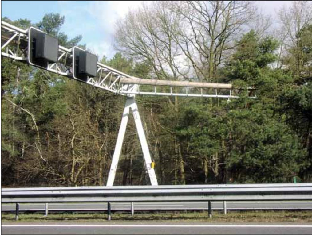
Figure 37. Photo. Canopy crossing installed in permanent signage fixture (Credit: Tony Clevenger).
