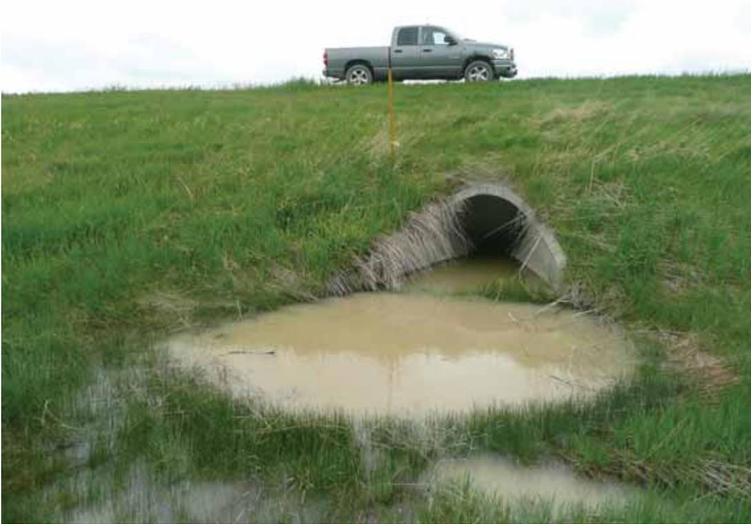
**Figure 58. Photo. Flooding in front of tunnel due to improper drainage design (Credit: Tony Clevenger).**
