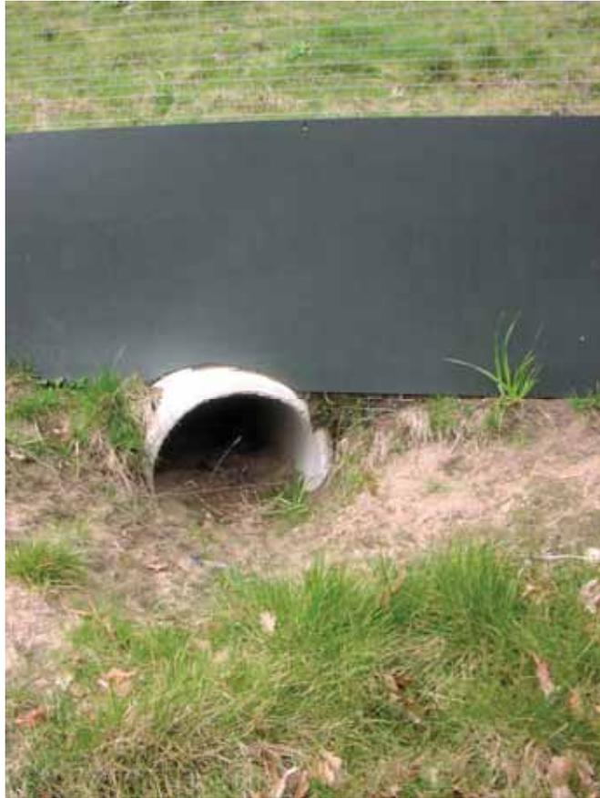
**Figure 56. Photo. Drift fence for amphibians and reptiles (Credit: Tony Clevenger).**
