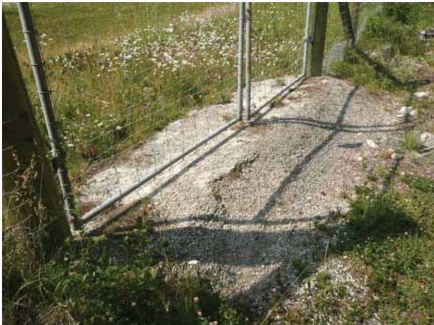
**Figure 66. Photo. Concrete base of swing gate to prevent animal digging under wildlife fence (Credit: Tony Clevenger).**
